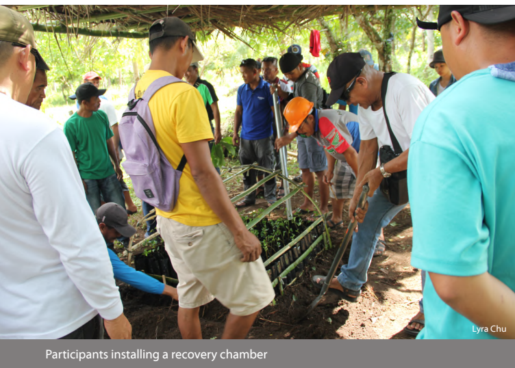
Participants constructing a low-cost nursery
