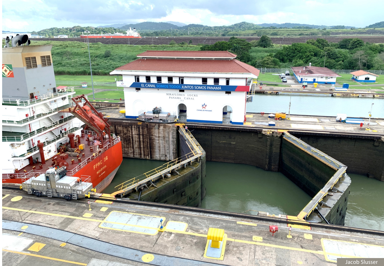
A ship being lowered to the elevation of the Pacific Ocean in the Miraflores Locks.
